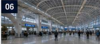
INTERNATIONAL AIRPORT Dammam, KSA Advanced ventilation systems for optimal passenger comfort.
