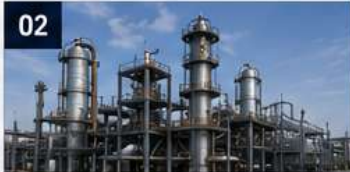
INDUSTRIAL PLANT Jubail, KSA High-performance ducting solutions for a large-scale industrial facility.
