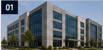
COMMERCIAL OFFICE COMPLEX Riyadh, KSA Complete HVAC duct system for a premium office complex.
