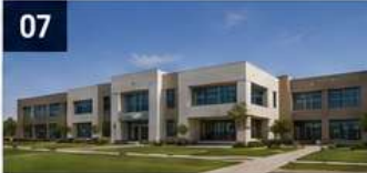
EDUCATIONAL INSTITUTION Riyadh, KSA Safe and efficient HVAC systems for learning environments.
